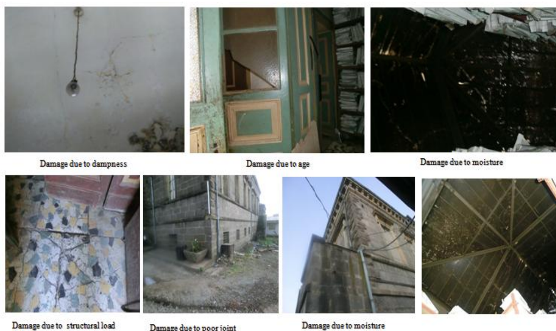
Fig 2. Some damaged parts of old Bank of Abyssinia (source: Author)
